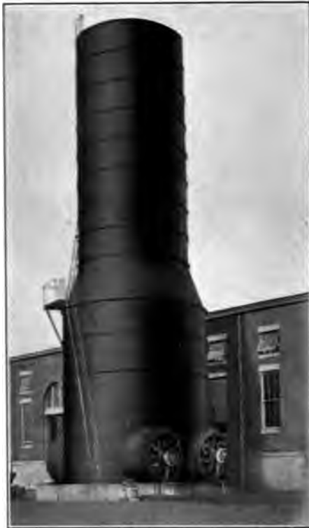
FIG. 76.—Worthington forced-draft cooling tower.
